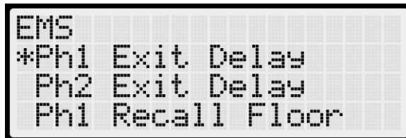
Figure 323: EMS Menu – Ph1 Exit Delay, Ph2 Exit Delay, Ph1 Recall Floor
